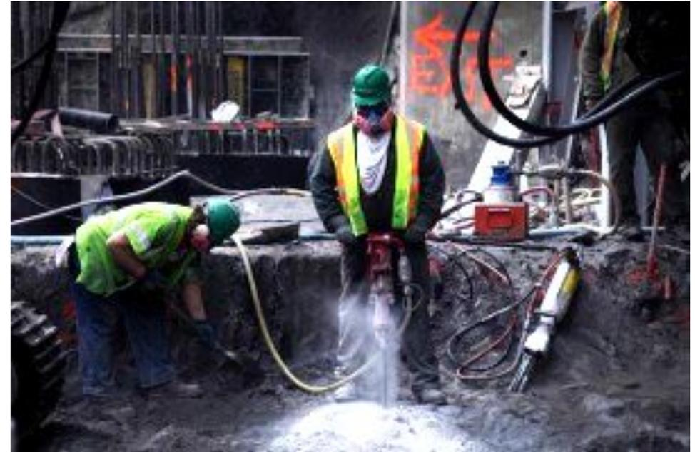
**Wear ear protection** both when you are exposed to noise and when you do not use the machines directly but they are used by other workers on site!
