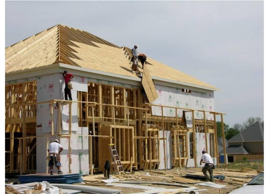
**Above 2 meters** it is necessary to set up adequate **protection measures!**
