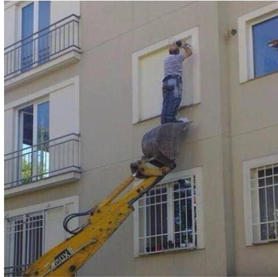
Use the **telescopic lifts** with the appropriate cabin and **wear a safety harness!**
