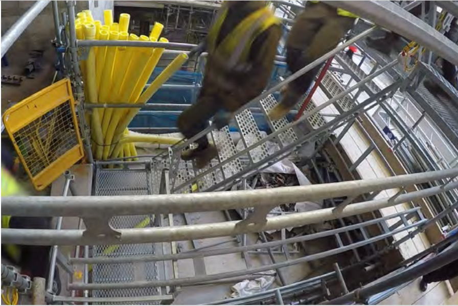
(a) First person of a group of four is on tread 3, with one other person on the stair and one more on the half landing.
