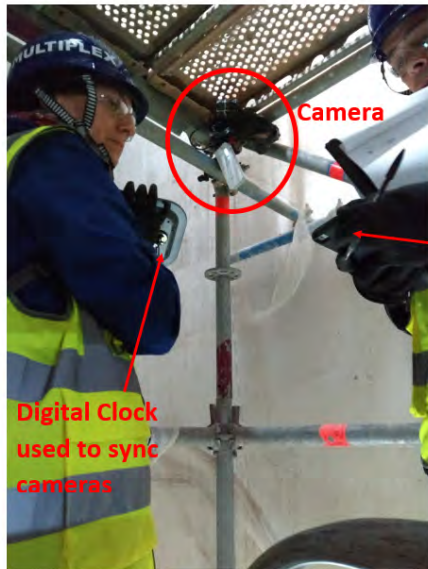
(a) Camera being set up on the stairs.
