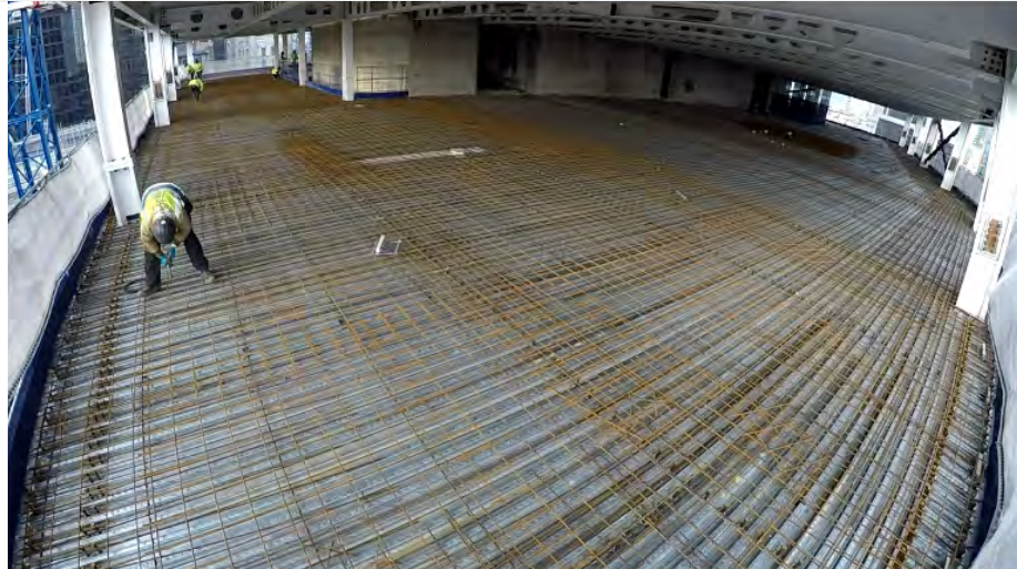
Figure 50. Worker installing rebar.
