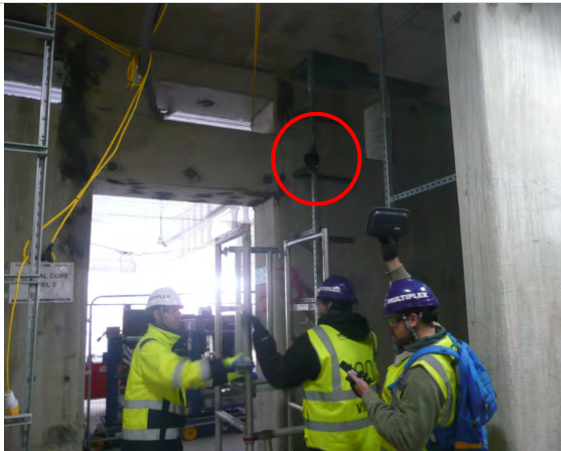
Camera (11) being set up on Level 4 in core.
