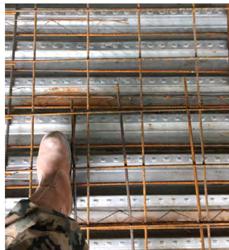
(b) Metal decking with rebar.
