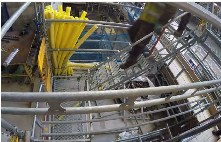
(a) Start of a group of two on the final flight; the first person is on tread 3, with one other person on the stair and one more on the half.
