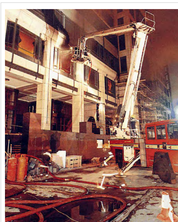
The Broadgate Phase 8 fire, London, UK 23 June 1990 [10]
