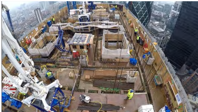
(a) View of top deck of slipform.
