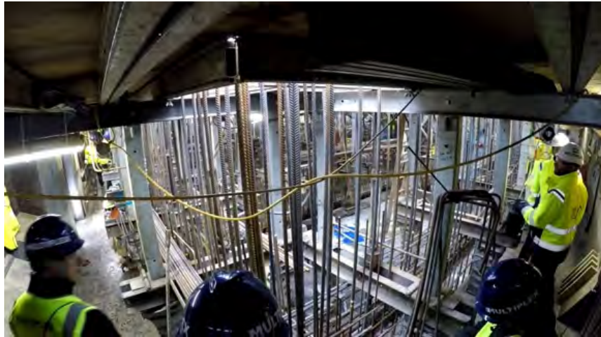
Figure 12. Typical conditions within the formworks.
