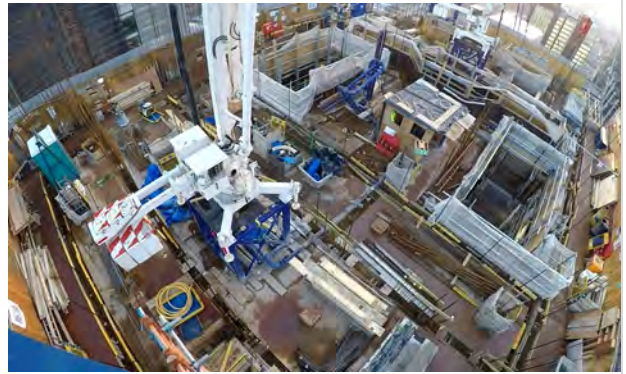
View from camera (23) in slipform.
