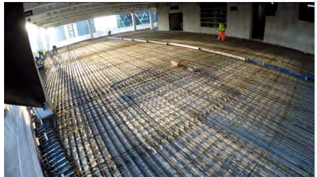
View from camera (7) on Level 7 on floor.
