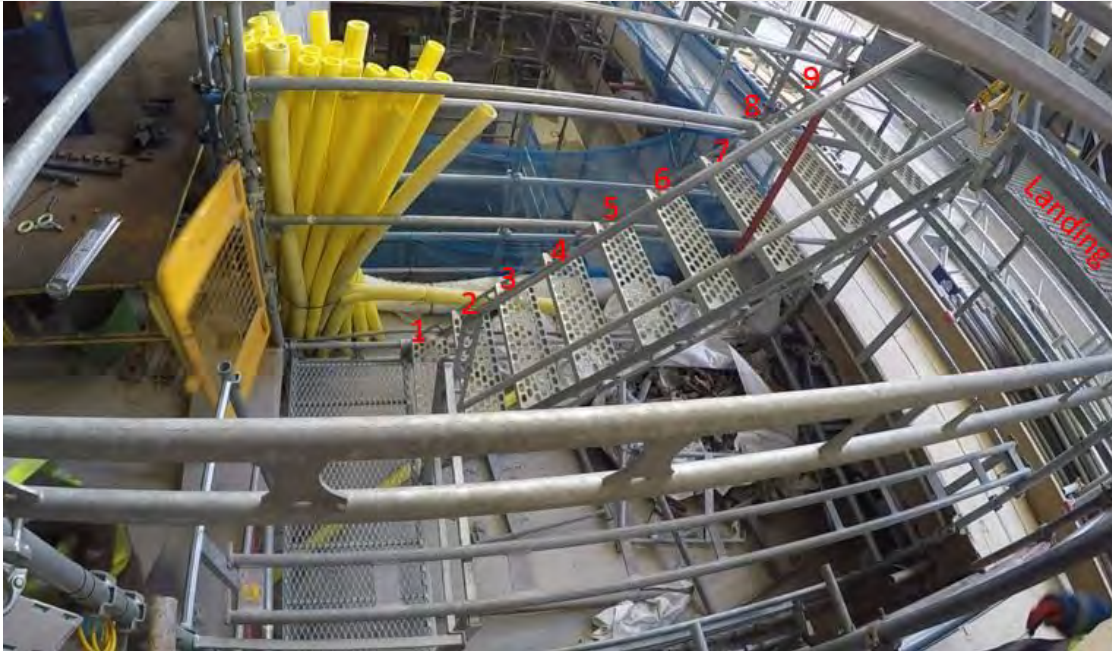
Figure 61. Stairs in Trial 2 used to collect stair usage data.
