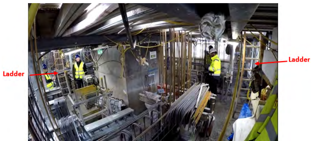
Figure 13. Two ladders connecting levels of the jumpform at 100 BG.
