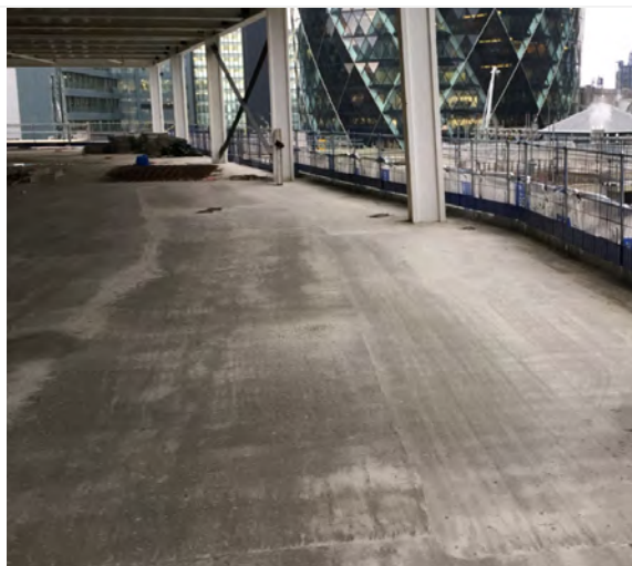
(a) Concrete surface.
